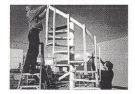
Before attaching the handrail, screw attach the lower newel baluster and newel base.
